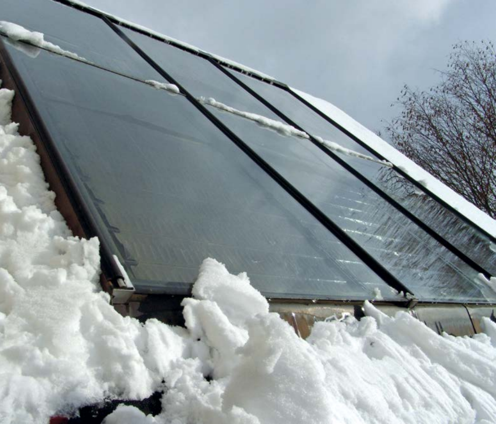
Stressing of the PV module
